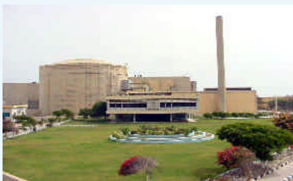
▲ Karachi Nuclear Power Plant (KANUPP), a 137-MW e Pressurized Heavy Water Reactor (PHWR)
